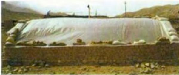
Poly-sheet secured with bags filled with mud, placed on the roof and on the side walls
